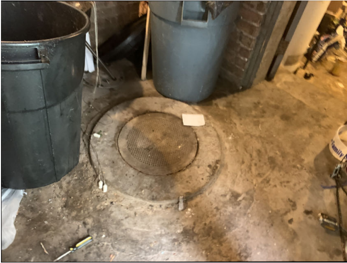
front catch basin
