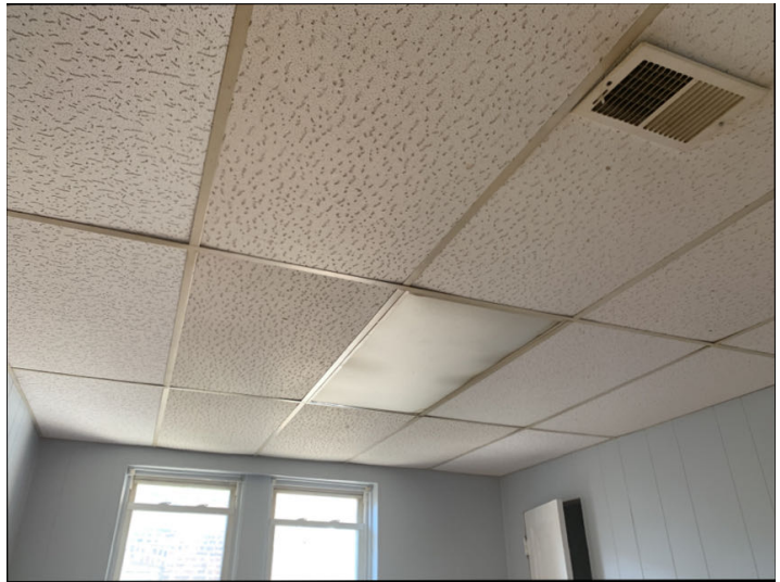
1E2 drop ceiling
