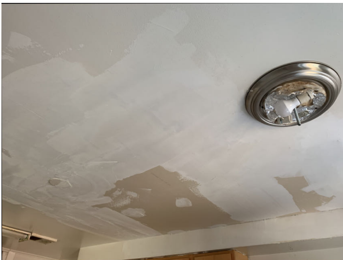
2D repaired ceiling
