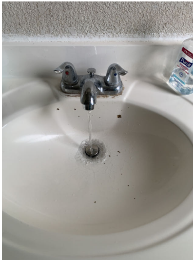
2W loose faucet and damaged basin
